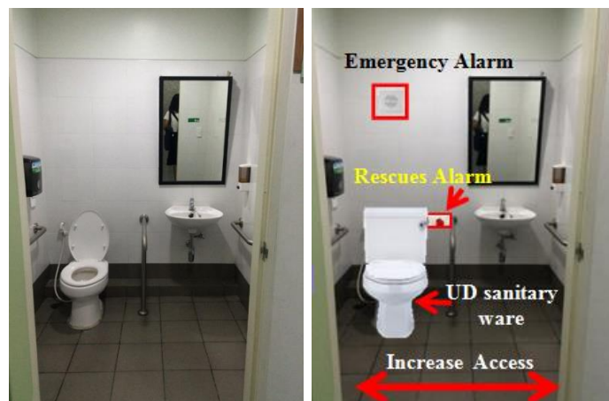
Figure 5: illustrates the changed sanitary ware as well as installed disabled equipment and emergency alarm
